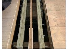
While removing the timber flooring to the Sanctuary area we noticed that the Tabernacle was supported by it's own pillar in order to take it's weight. This made sense, since the Tabernacle is over 400kg. We therefore, dug down 200mm and created a concrete base before building a strong pillar in the new and proposed location of the Tabernacle. This will hold it.
